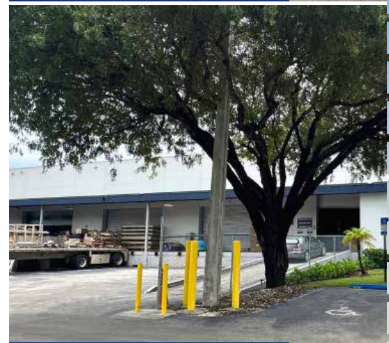
Oversized dock doors
